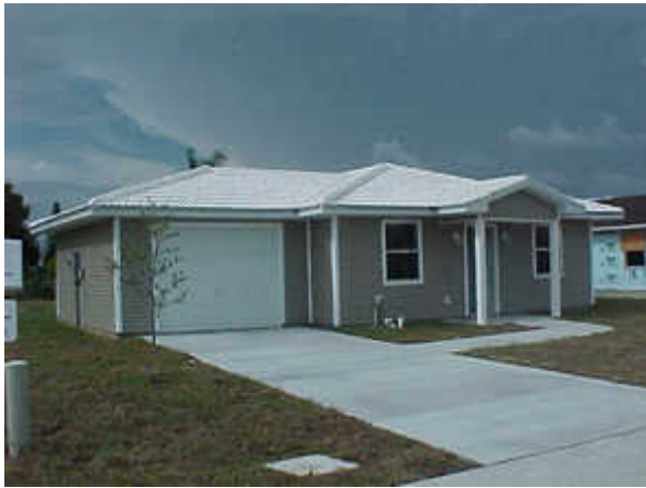
White s-tile roof home
