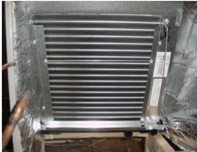
Slanted coil arrangement
