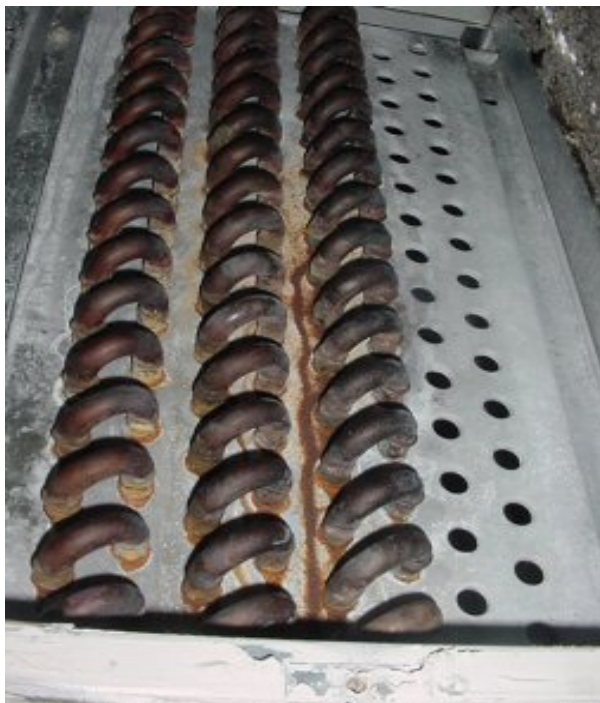
Figure 5. Coil U-bends
