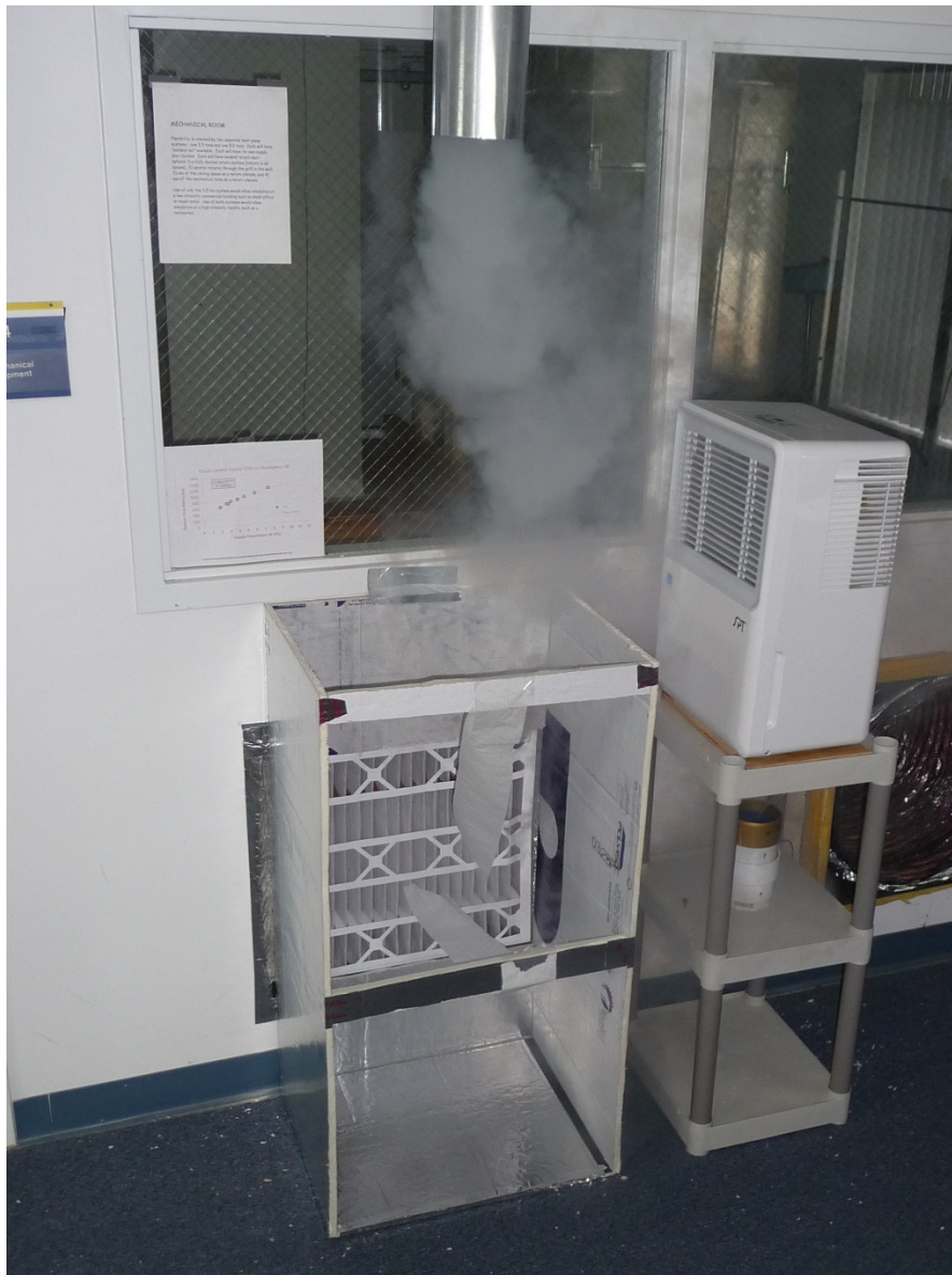
Figure 4. Fog injected into the OA intake shows Capture of OA at 60cfm into central return during the central system's lowest stage of cooling and low system flow rate. Tissue paper indicates air flow direction from room into return.
