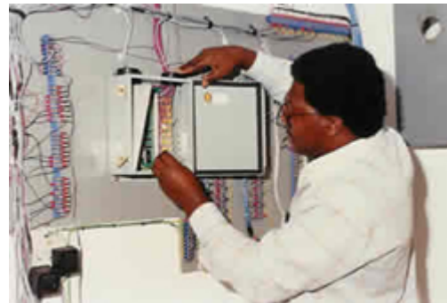
Figure 17. Engineer Elvis Gumbs adjusts thermocouple arrays
