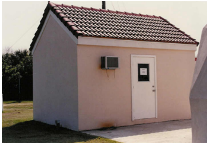
Figure 11. The Dow prototype after retrofit with red concrete tiles.
