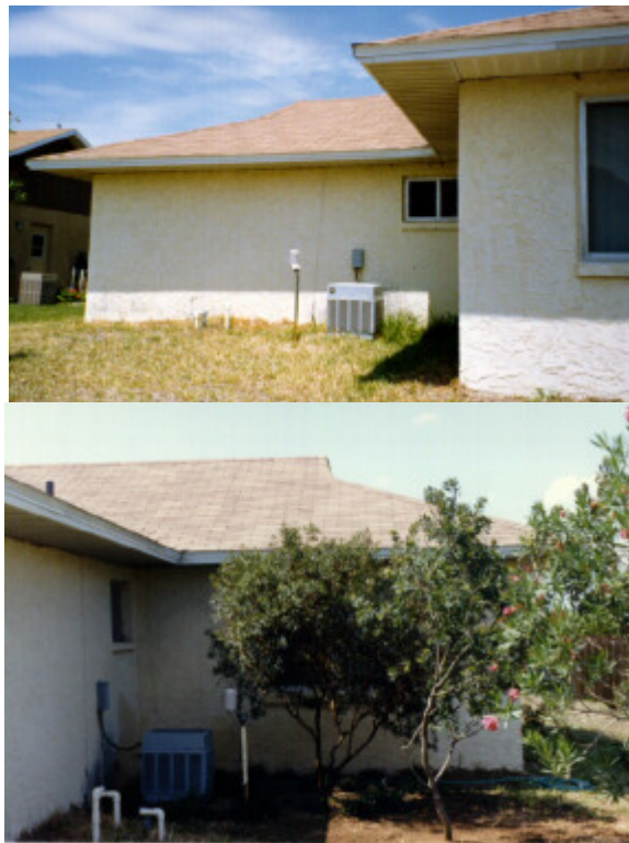
Figure 4. West-facing condenser at site 1 prior to landscaping (top). Final appearance after tree planting (bottom).
