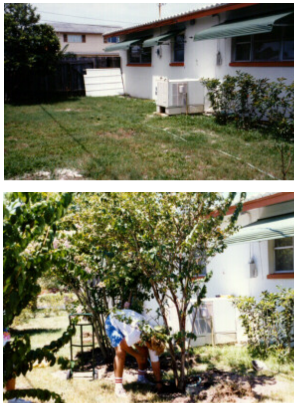
Figure 8. West-facing AC condenser shading at site 3 before landscaping (top). Planting of four Crape Myrtles for shading (bottom).
