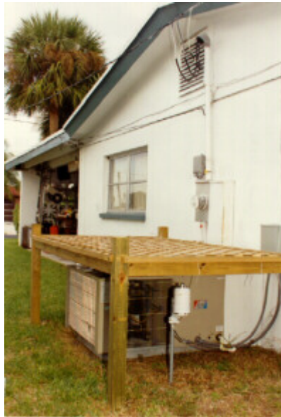
Figure 7. Trellis shading device built over the condenser at site #2. The packaged unit draws air through inlets on each side and exhausts air horizontally from the house.
