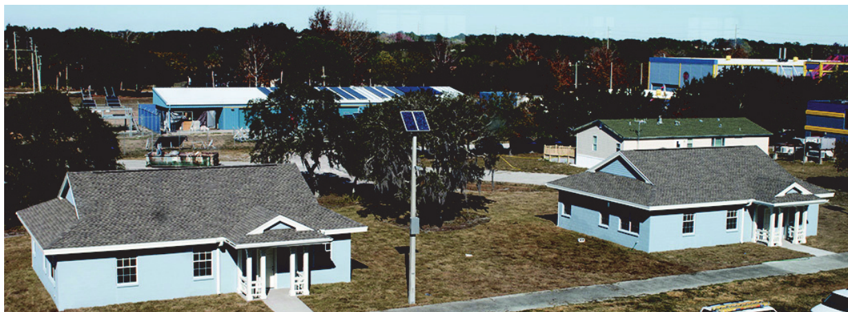
Figure 1 Side-by-side FRTF buildings at FSEC in Cocoa, Florida.
