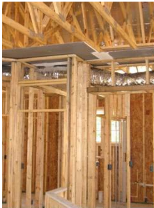
Figure 2. Fur-down chase after rough framing.
