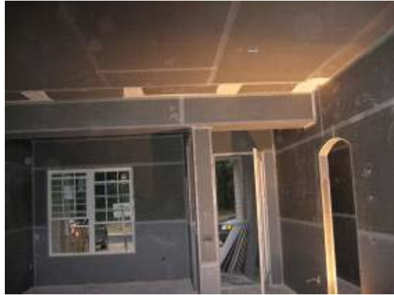
Figure 17. Free-hanging chase across an open space. Note separation of space accentuated by chase.
