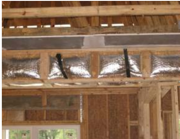
Figure 23. Finish framing for chase.
