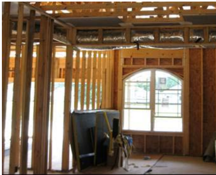
Figure 28. Chase sides and bottom installed.
