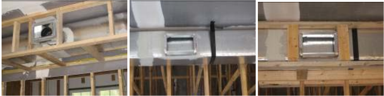
Figure 29-31. (Left to right) Connecting flex duct to a trunk line for a supply run-out results in a wide chase. Instead, a supply outlet constructed from a duct board box can be directly affixed to the trunk. This permits construction of a much narrower chase.
