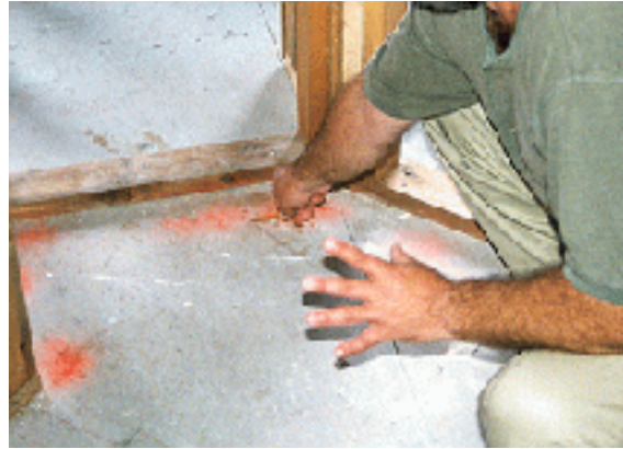
Figure 19. Paint tags alerting crews to the location of the proposed chase.
