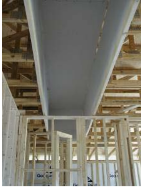
Figure 1. Fur-up chase installed after rough framing.
