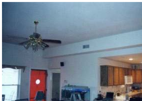
Figure 8. A fur-down chase used for architectural detail.
