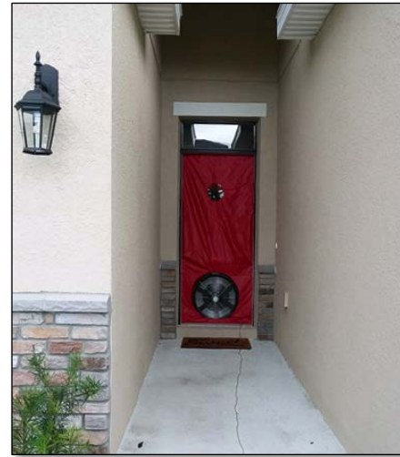
Figure 1. Blower door set-up at study home.
