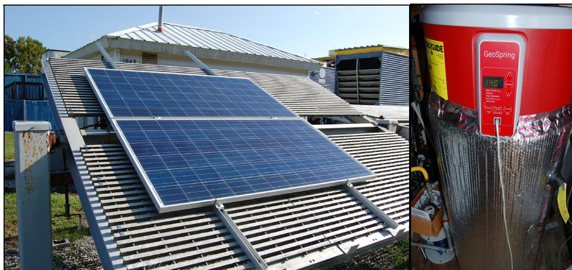
**Figure 1: PV modules (310 Watts each) and 189-Liter HPWH shown with added insulation**
