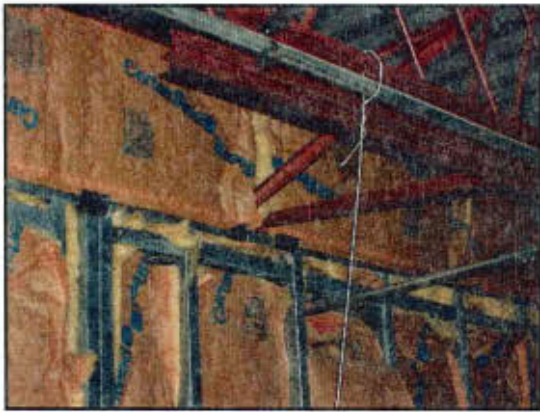
Figure 36. Wall insulation above ceiling
