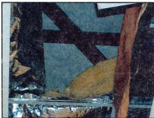
Figure 4. Missing air barrier & insulation that had been moved to gain access to attic
