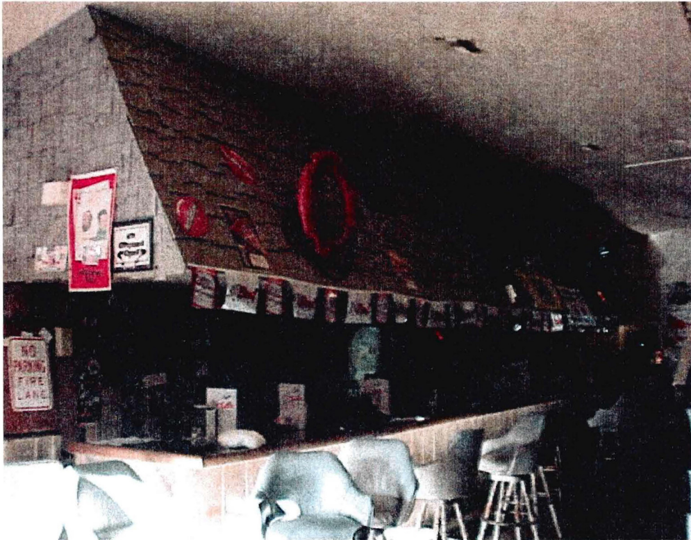
Figure 3 Ceiling over bar area was very leaky and poorly insulated.
