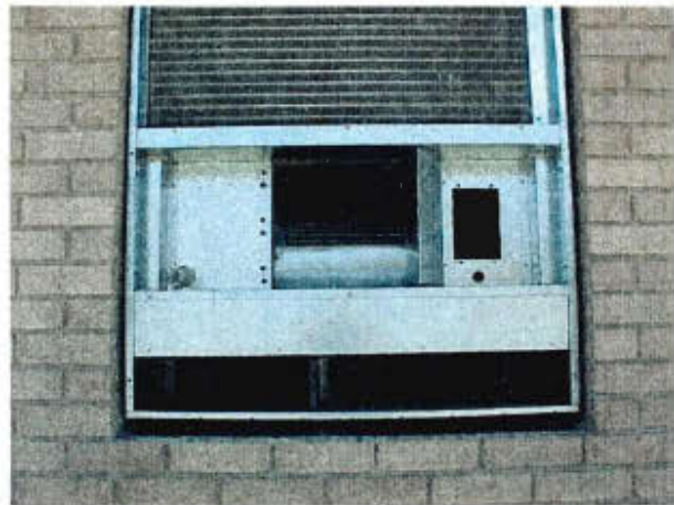
Figure 15 Exterior view of PTHP unit with grille assembly removed. Approximately 1 inch of clearance exists between the unit and the wall.
