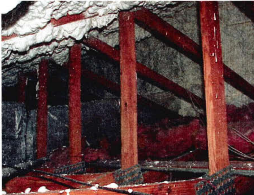
Figure 4. View of attic air / thermal retrofit with void in original batt insulation shown at the bottom of picture.
