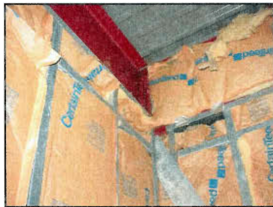
Figure 37. Insulation fallen from beam.
