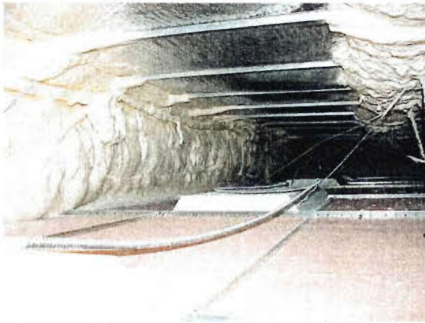
Figure 16 Finished air sealing above the t-bar ceiling.
