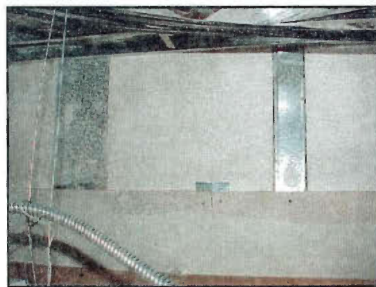
Figure 5. Incomplete air barrier at connection of wall assembly to ceiling
