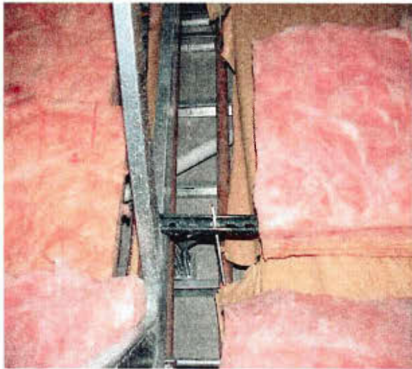
Figure 14 Typical insulation void approximately 25% to 30%.
