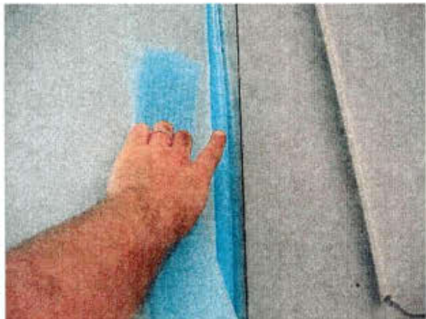
Figure 19 Gasketing material placed between the PTHP and the wall to create a seal.
