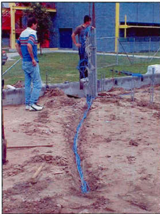
Figure 2. Thermocouple wire being installed under slab.
