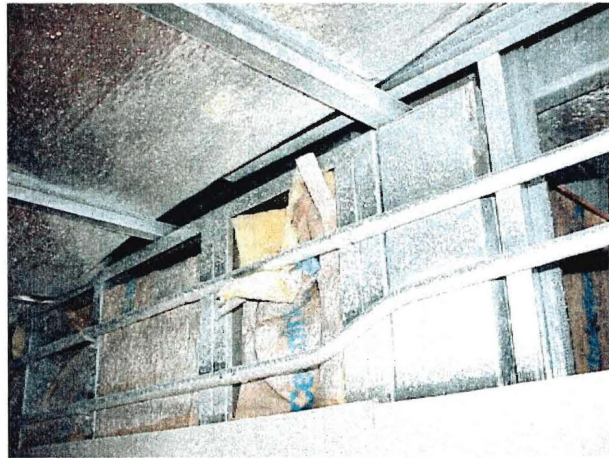
Figure 13 Incomplete air barrier over t-bar ceiling.
