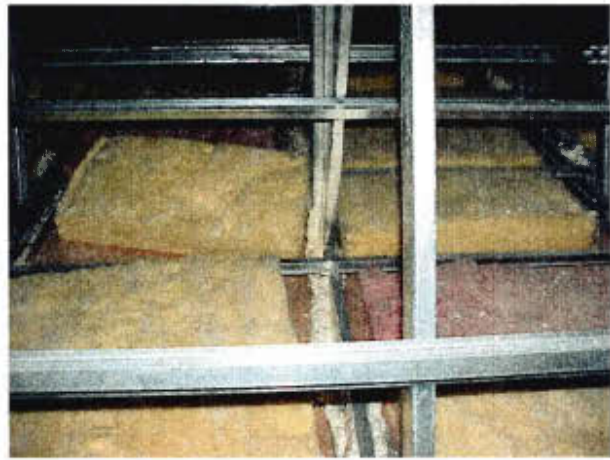
Figure 17 Attic space after foam was installed. It can be seen along the bottom of the truss.
