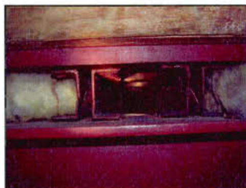
Figure 35. Air leak pathway where metal truss sits on top of structural beams.
