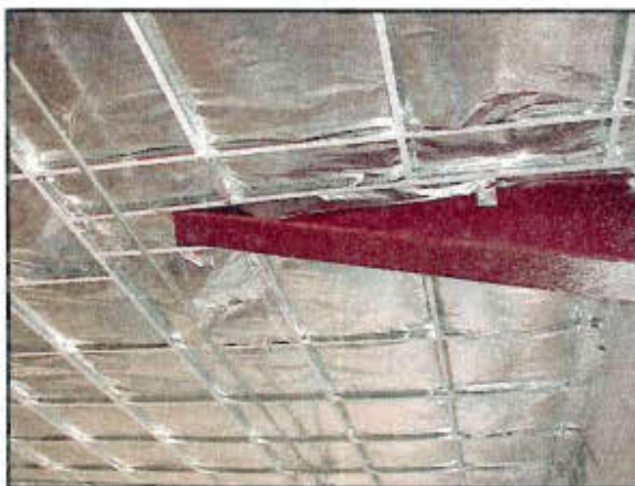
Figure 6. Metal grid system covered with radiant barrier acting as air barrier. Numerous gaps exist, especially at penetrations of the grid assembly.
