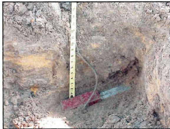
Figure 3. Soil moisture sensor being installed 12 inches below slab.
