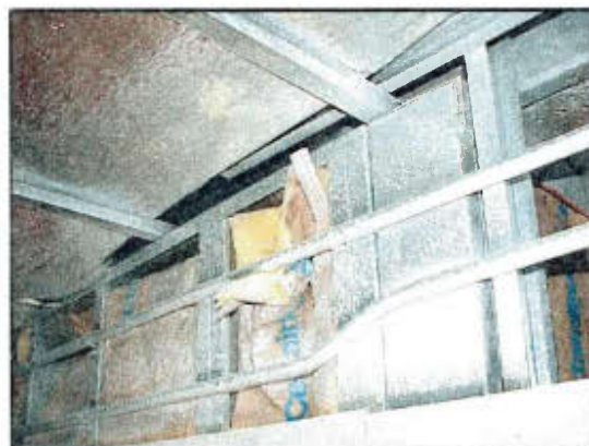
Figure 7. Incomplete air barrier over t-bar ceiling.
