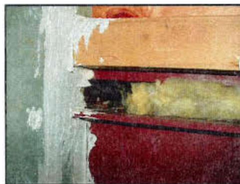
Figure 34. Gap above structural beam
