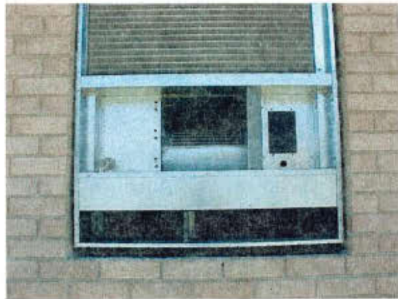
Figure 9. Exterior view of PTHP unit with grille assembly removed. Approximately 1 inch of clearance exists between the unit and the wall.
