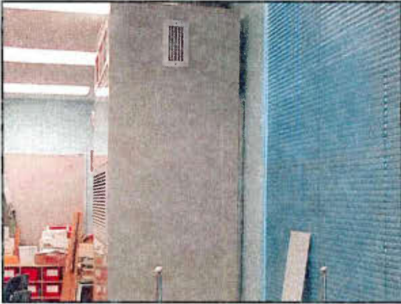
Figure 8. The interior decorative trim has been removed to show the space between the unit and wall. This space is approximately 1 inch.
