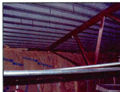
Figure 33. Ceiling space showing gap at roof deck to wall intersection.
