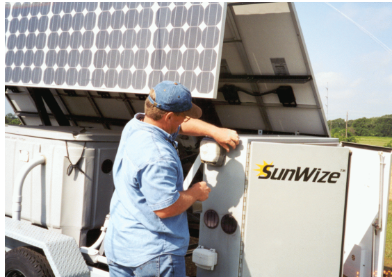
Figure 6 Repairing power outlet cover in Denton unit
