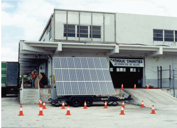
Figure 15 Mobile PV generator at a distribution center
