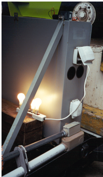
Figure 5 Invertor load test
