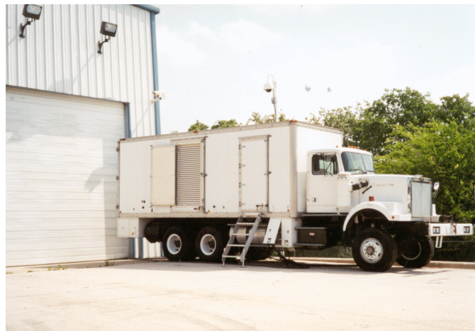
Figure 12 50 kW diesel generator in Denton, Texas
