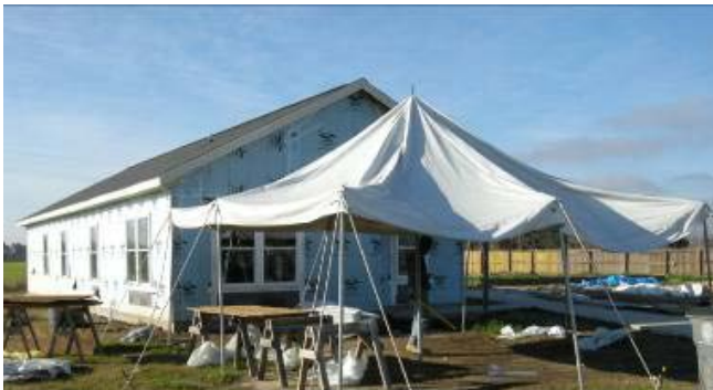
Figure 6. Baton Rouge Habitat 30% affordable demonstration house.
