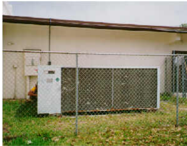
Figure 3. Forty-ton air cooled liquid chiller.
