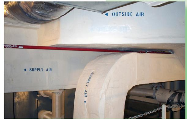
but ineffective humidity control. Fan AUTO control yields better RH control but does not provide reliable ventilation. **Solution:** install a system which separately conditions ventilation air. We recommend that a DOAS with dedicated OA distribution provide the necessary ventilation while also effectively stripping water vapor from the OA. A DOAS with dedicated air distribution also reduces the potential for overcooling and the need for reheat.
