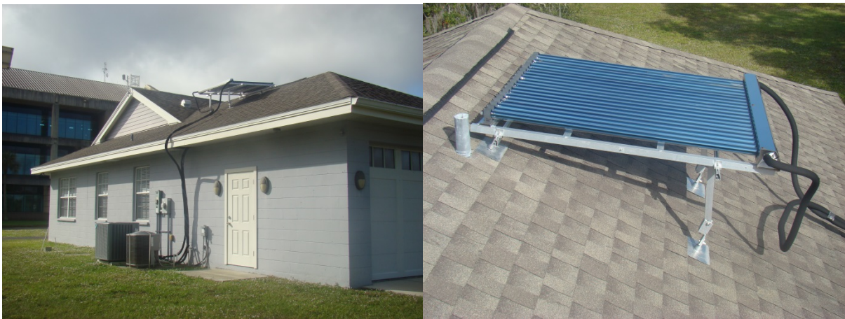
Figure 2 Solaire Collector installation
