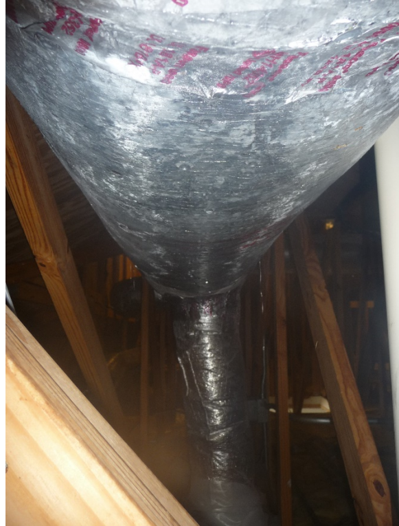
Figure 18. Close view of finger swipe on jacket surface shows light condensation on section within the largest circle shown in Figure 17 (9/18/20).
