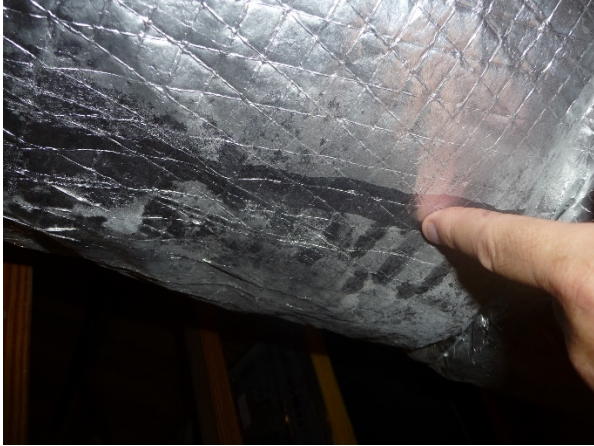
Figure 18. Close view of finger swipe on jacket surface shows light condensation on section within the largest circle shown in Figure 17 (9/18/20).
