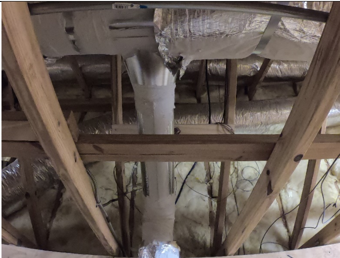
Figure 3. A shiny new duct branch “B1” is shown here during installation in June 2019.
