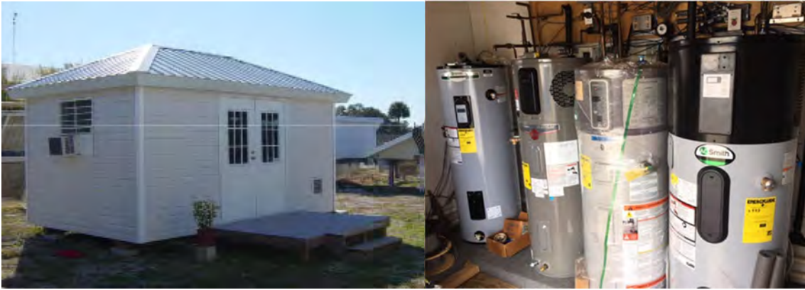
Figure 2. FSEC's hot water research test facility.
