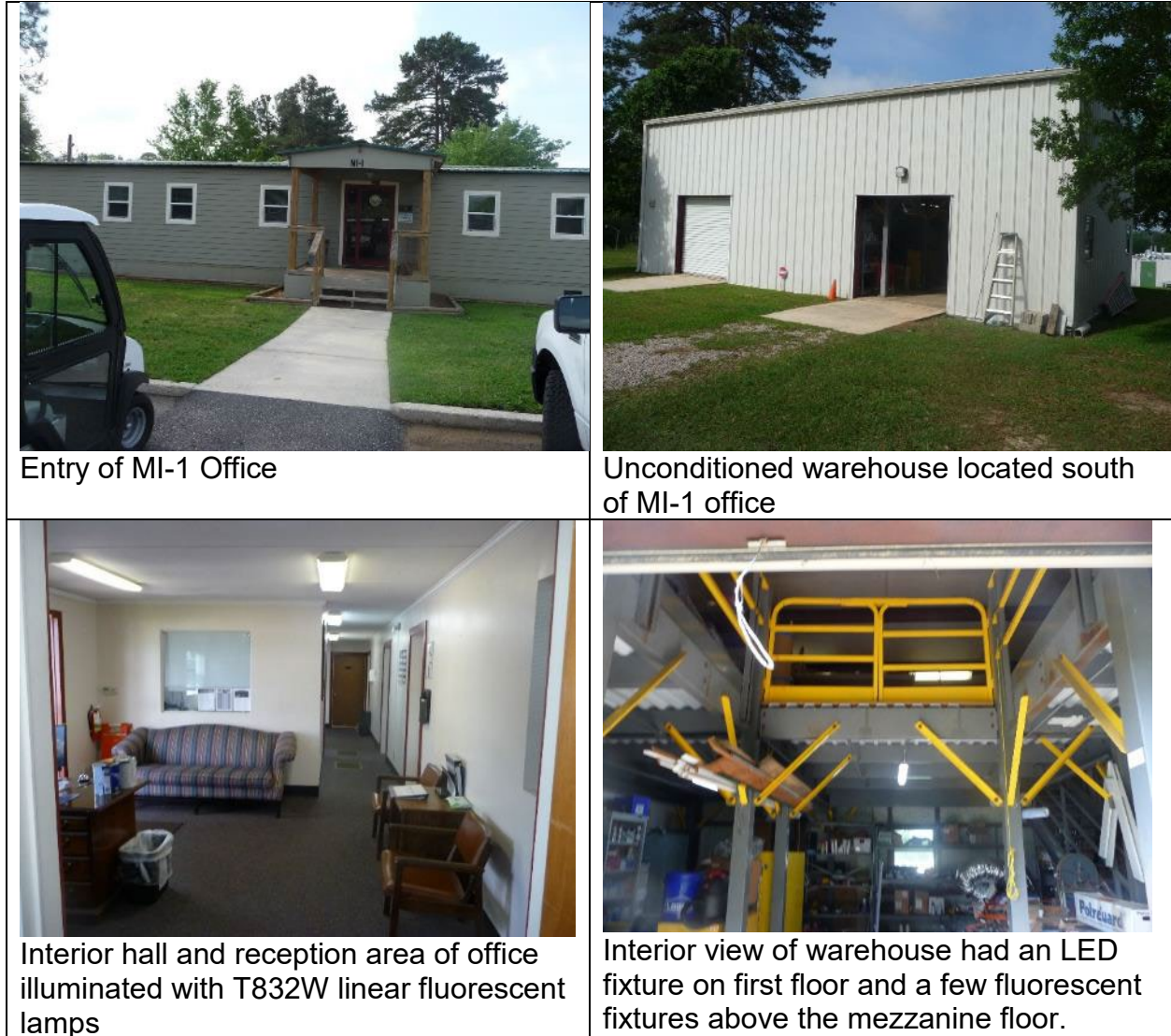
Figure 35. MI-1 Maintenance Office.
