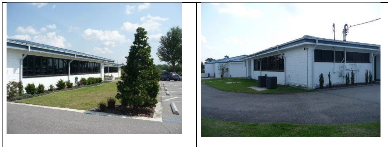
Figure 8. Left: Front side of buildings facing southwest with west building dominantly shown. Right: Back side facing northeast and northwest side with new power mast and electric meter. Two 5 ton Goodman heat pumps located outside the west building.
