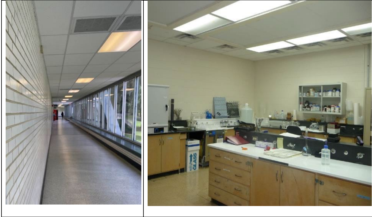
Figure 33. Left: Walkway connecting labs with lights controlled by occupancy sensors; Right: Example of a laboratory work space.
