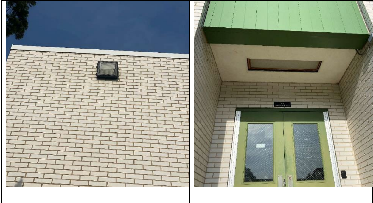
Figure 32. Left: Exterior wallpack; Right: Overhead entry lamp.
