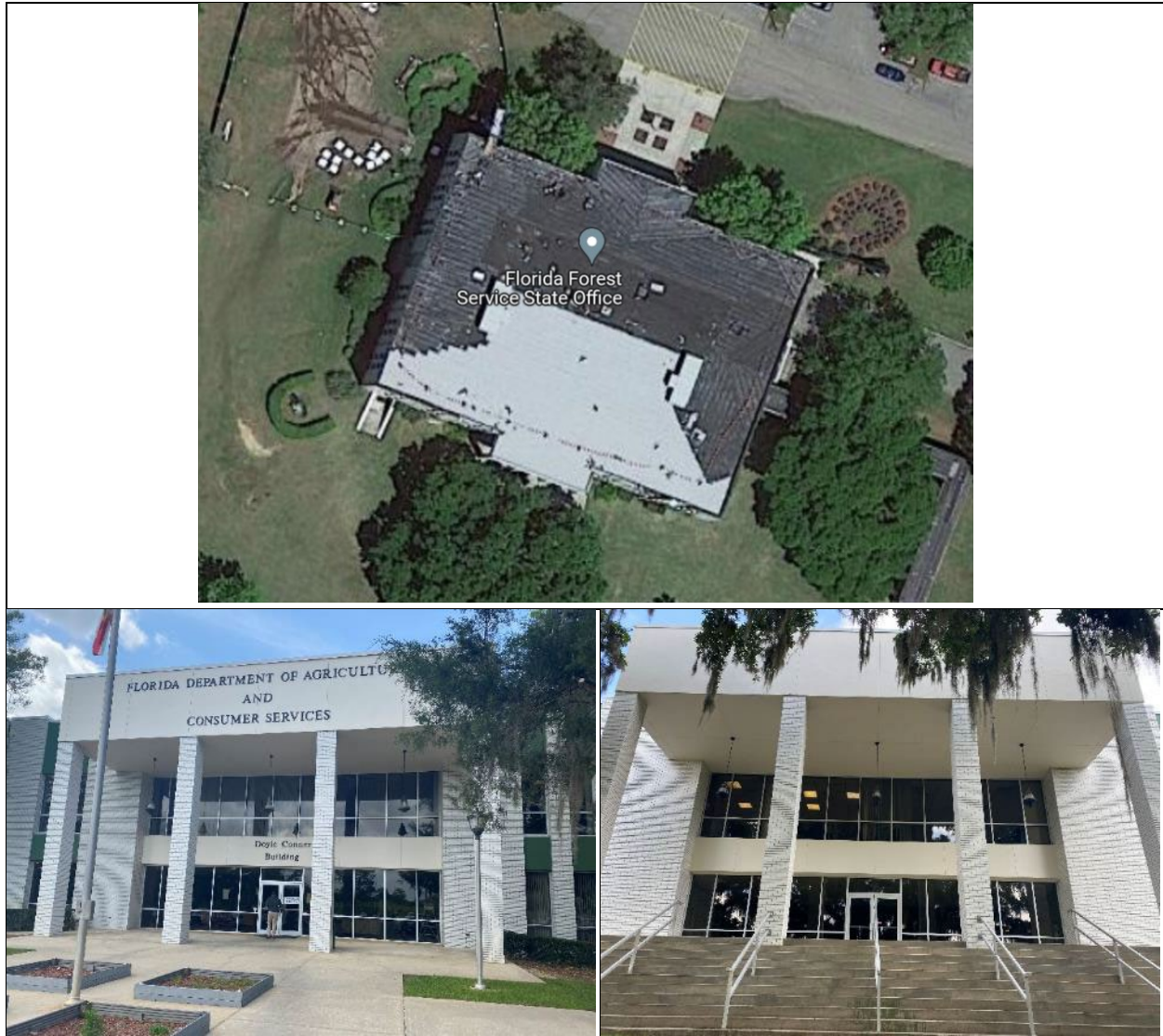
Figure 25. Conner Administration Building.
