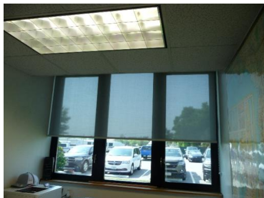
96ft 2 office with daylighting and a 4-lamp T8 fixture
