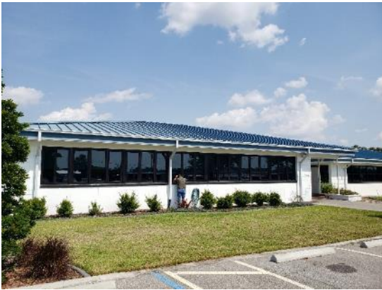
Southwest side of west office building.
