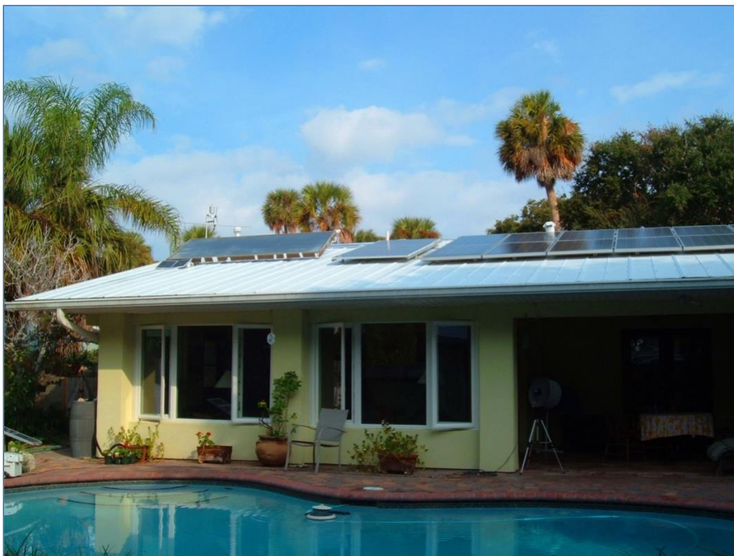
Figure 3: Home in Cocoa Beach: Solar hot water, PV pumped pool and 6 kW PV system.
