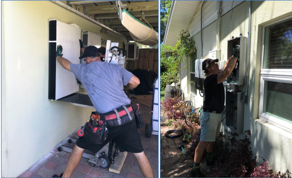
Figure 4: Installation of two Tesla Powerwall 2s on 22 May 2019
